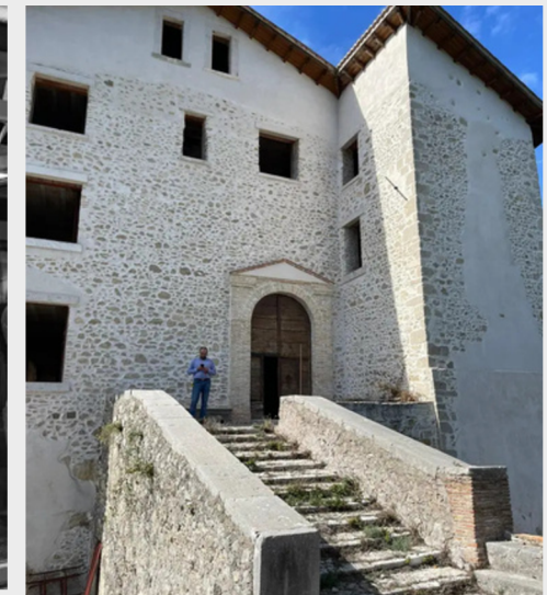
Site visit for measurements at a castle in Riofreddo, Italy
